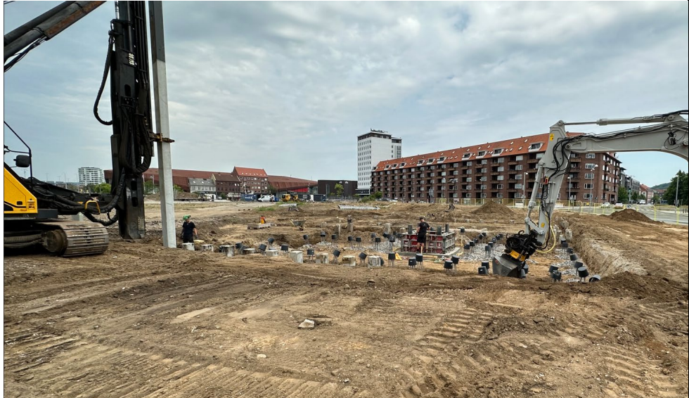
June 2023 – works on S1 and S2 project – sold part
