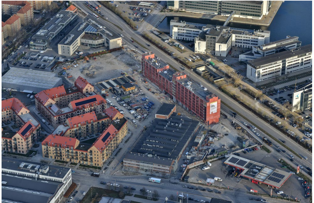
Status november 2023 – Student House
