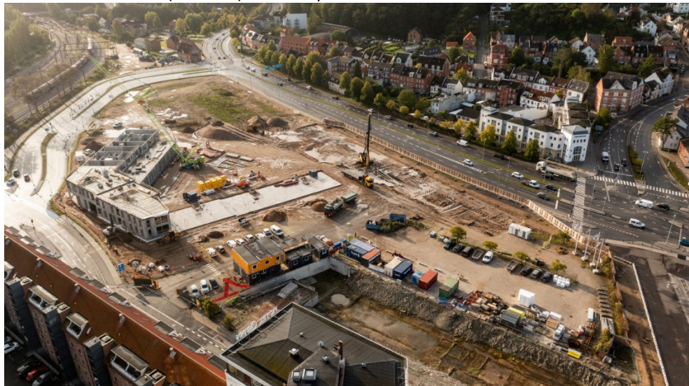
September 2023 – on going construction of residential structure – sold part of project. Pile foundation of S6 (machine) 50% complete.
