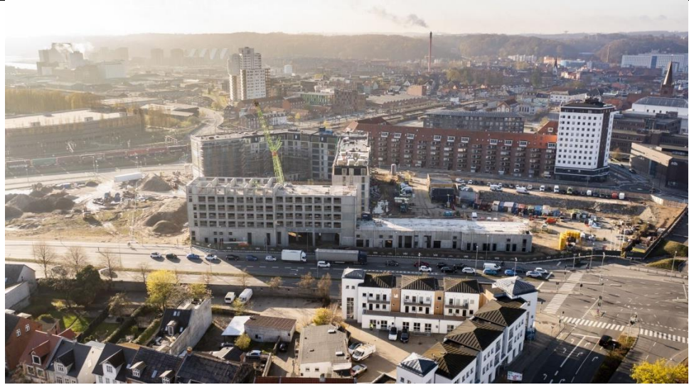
January 2024 – GHV 1+2 and Micro Living under construction
