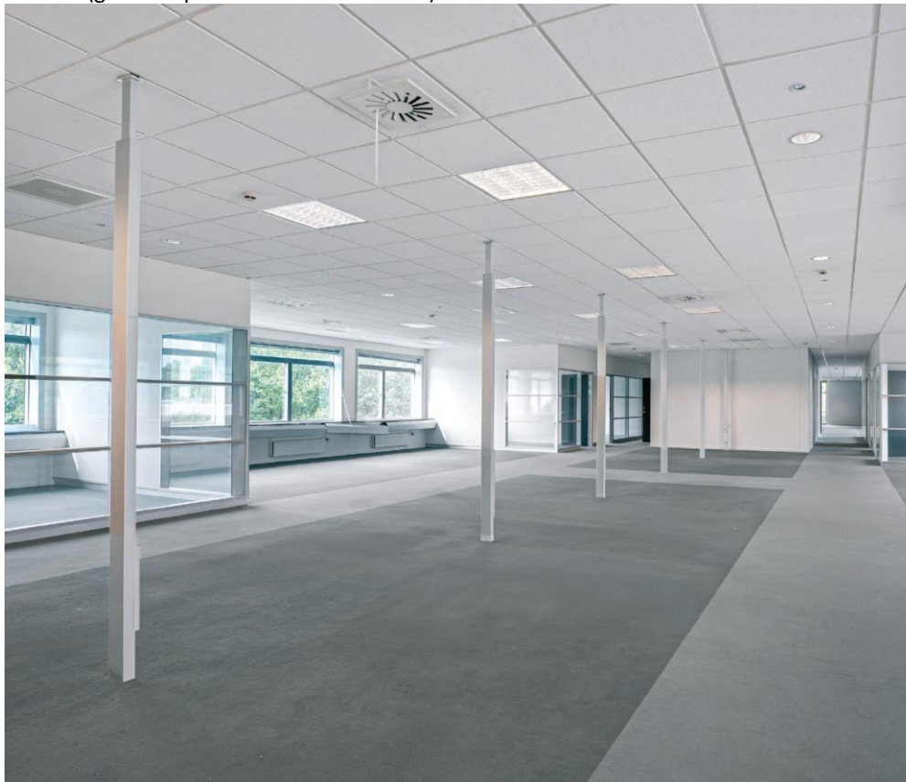
Current (good shape but to be modernized):
